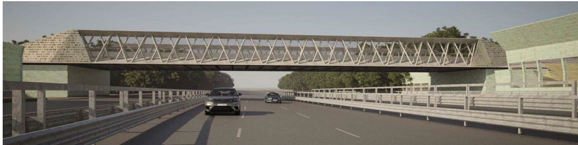
VIA BENAZZA OVERPASS (CGI)
