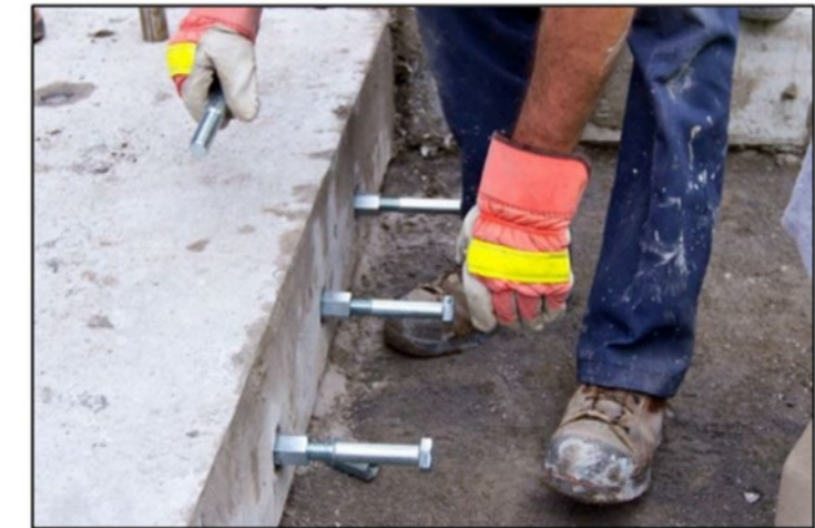
Restoring Tie Bars
